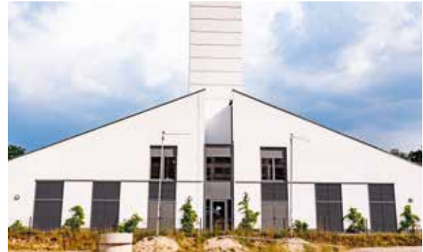
Co-generation plant at the "52 Grad Nord" development project in Berlin
